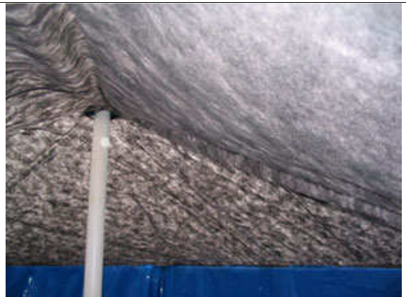
Pole supporting insect proof roof
