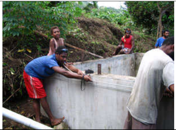
Installing the wire straps around the tank to prevent further movement
