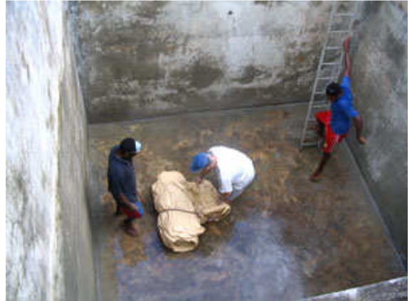
Time to install the liner
