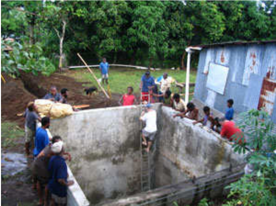
A trench dug down to the outlet pipe
