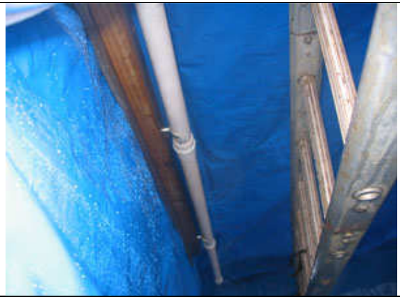
The pump extracts water from the bottom of the tank (safer for the liner than the usual method of lowering buckets attached to sharp sticks)
