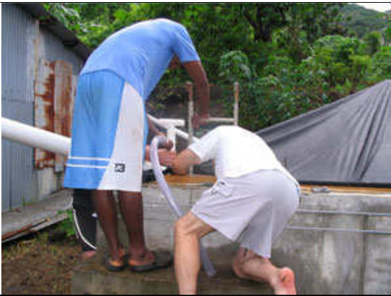
Installing the pump Note the insect proof screen over the tank
