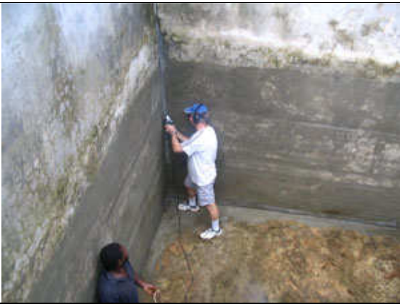
Craiger sanding the repairs to remove any rough edges
