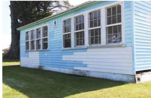
**Thursday:** Old style weatherboards are an interesting feature of this building – but a number have cracked and twisted over time. The worst ones are being replaced prior to painting.
