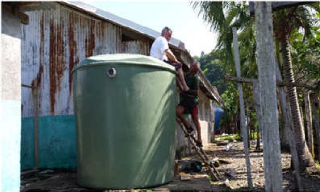
Kerry and Francois replacing some of the roofing iron and adding new guttering to feed the new 6000 L tank
