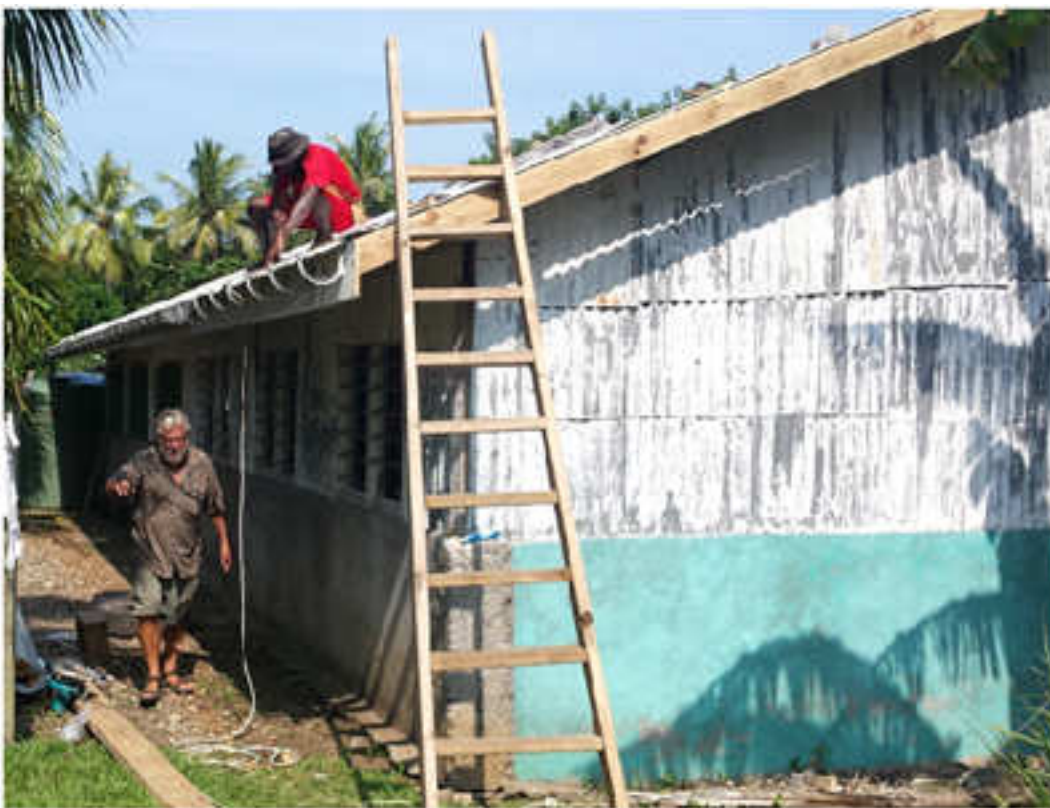
Kerry and Francois replacing some of the roofing iron and adding new guttering to feed the new 6000 L tank
