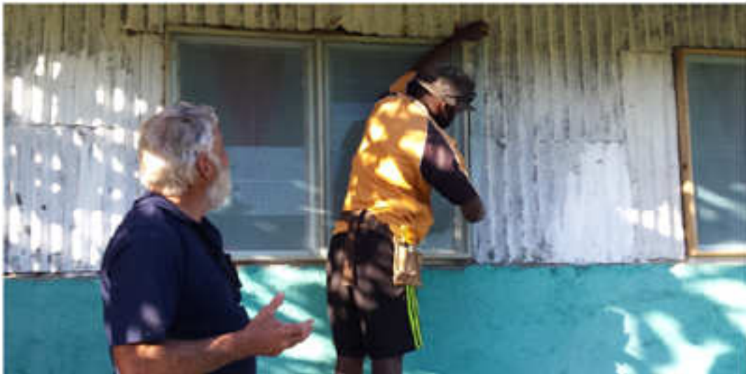
Kerry and Francois fitting Mosquito Mesh on the Dormitory Windows.
