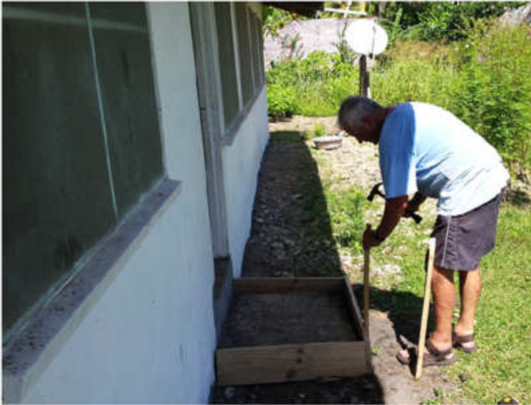
Dave preparing boxing for new concrete door step
