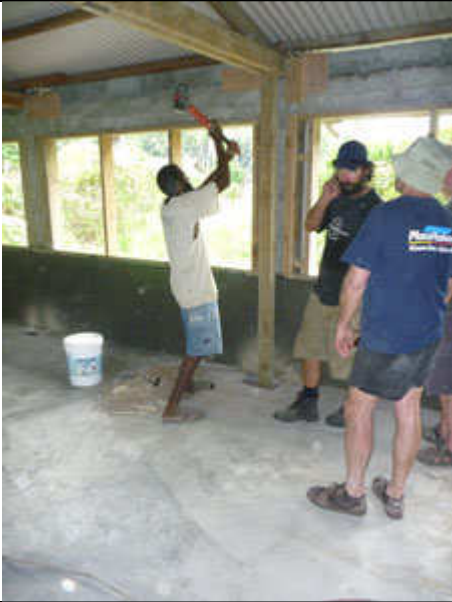
Two expert builders (Emile and Richard) arrive in the second week and install new timber columns to tie into the repaired trusses and the steel in the floor.
