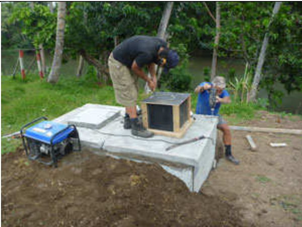
Thunder box installation. Once one tank is filled this tank is closed off and the seat moved to the other tank. When that fills the first tank is shovelled out as good useable compost
