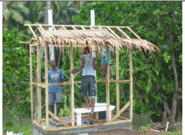
The thatched roof going on. A good thatch and bamboo walls last 25 to 30 years. The vertical pipes at the back remove the smell
