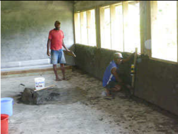
The walls freshly plastered
