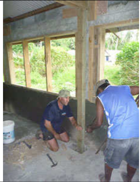
Two expert builders (Emile and Richard) arrive in the second week and install new timber columns to tie into the repaired trusses and the steel in the floor.
