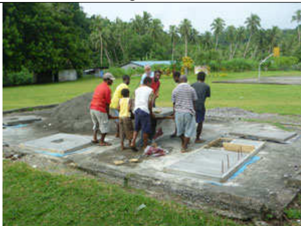
Carrying the slab – to the far end of the field
