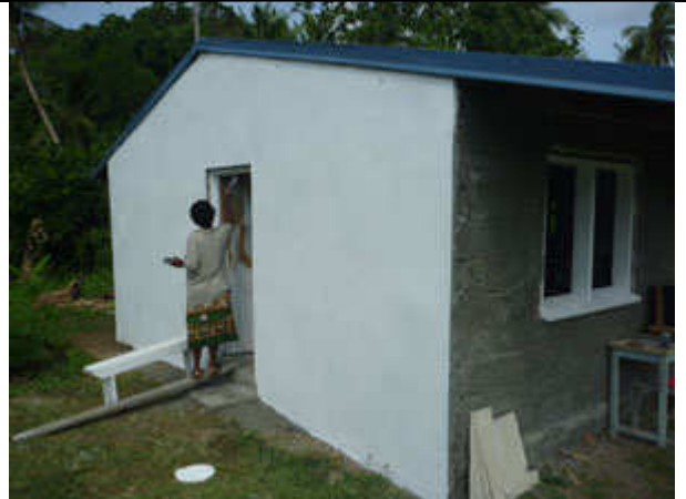
The other end wall complete after plastering, painting and flashing.
