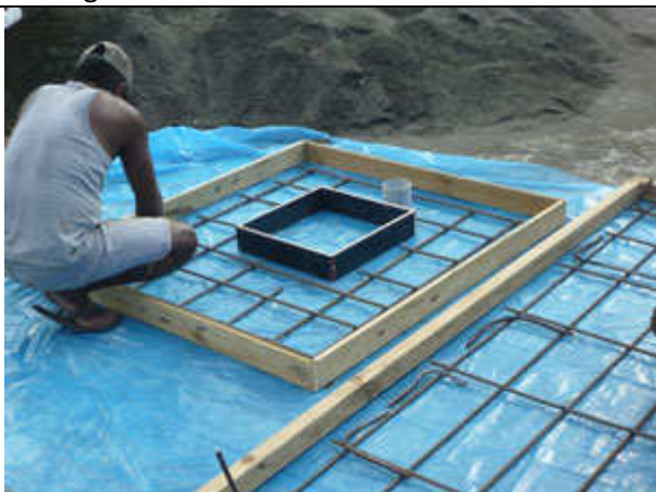
Building the framework
