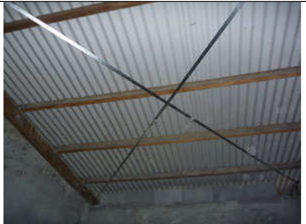
And adding roof bracing
