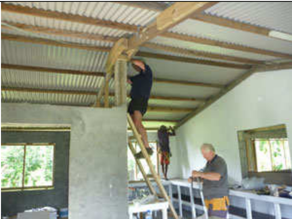
Fixing up the roof trusses
