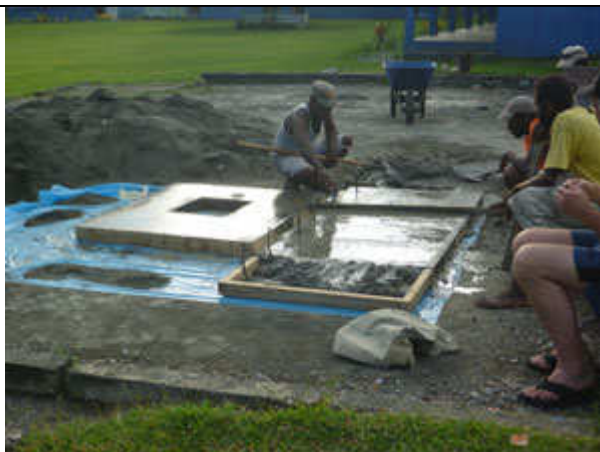
Pouring the concrete
