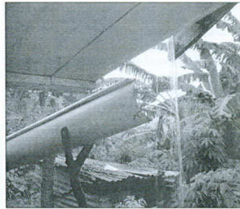
The hit and miss rain collection system on Tongoa as demonstrated at the school house. Early schooling is subsidised, but it is only the very rich and very able who progress to high school in Vila.
