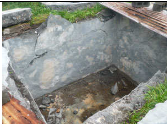
Damage ranged from cracks that emptied the tanks to total destruction
