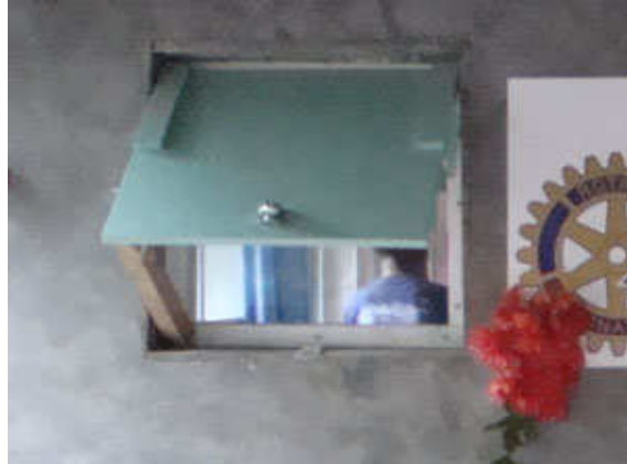
New hurricane shutter with mesh screen behind
