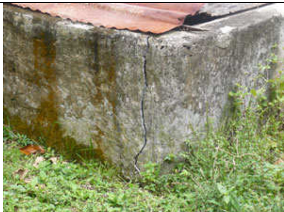
Damage ranged from cracks that emptied the tanks to total destruction
