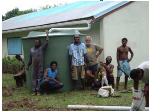
The tank installed by the Church (best roof in the village and at a good location to gravity feed by pipe back to the village)
