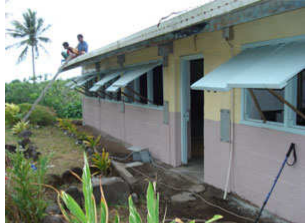
And during renovations
