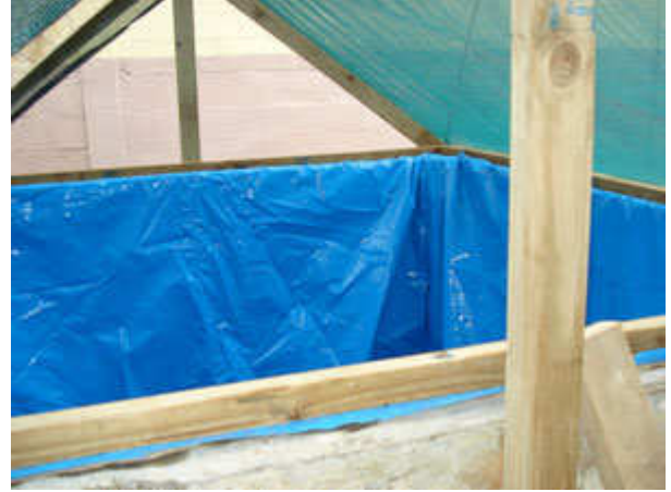
New Water tank liner
