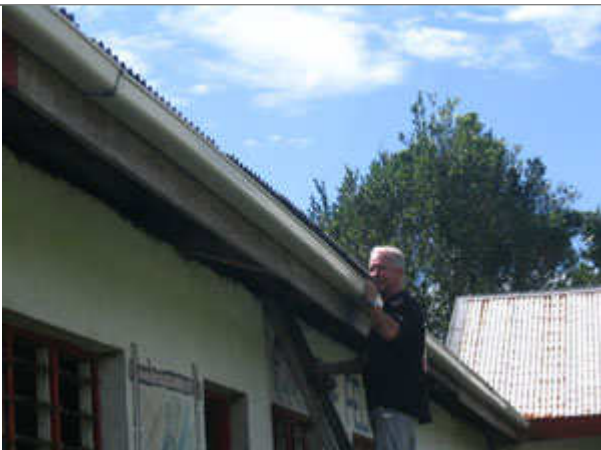
Craiger unblocking blocked gutters. One water tank – and plenty of rain – supplies the school
