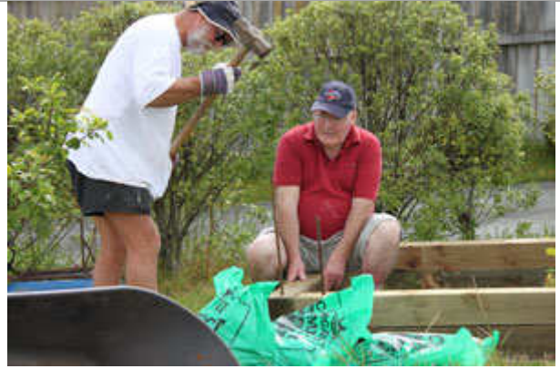
The timber is held together with metal rods inserted through drilled holes in the timber.
