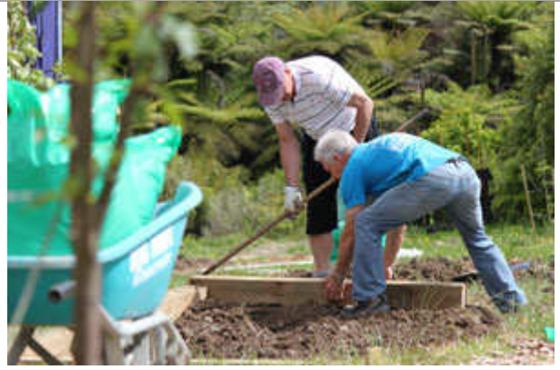
Noel and Craiger lining up the timber
