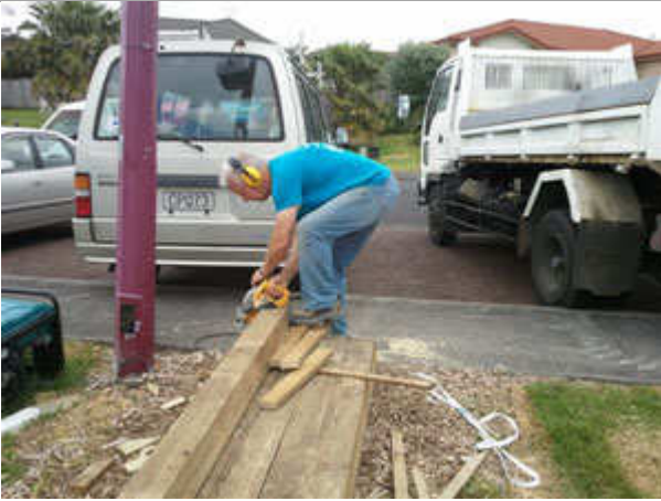
Craiger cutting the timber to size
