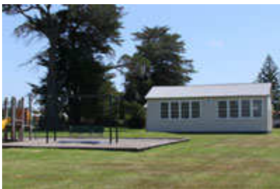
Girl Guide Hall Major Renovation
